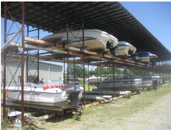
PHOTO: 13 COVERED OUTSIDE STORAGE FACING SOUTHEAST DATED 05/19/17 TAKEN BY TONY ESSA
