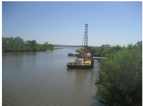
PHOTO: 20 COMMERCIAL SLIPS EAST DATED 05/19/17 TAKEN BY TONY ESSA
