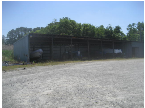
PHOTO: 14 COVERED OUTSIDE STORAGE FACING SOUTHEAST DATED 05/19/17 TAKEN BY TONY ESSA
