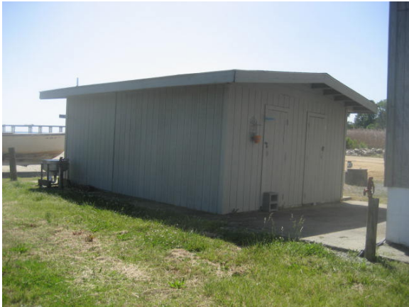
PHOTO: 3 REAR OF OUTHOUSE FACING EAST DATED 05/19/17 TAKEN BY TONY ESSA
